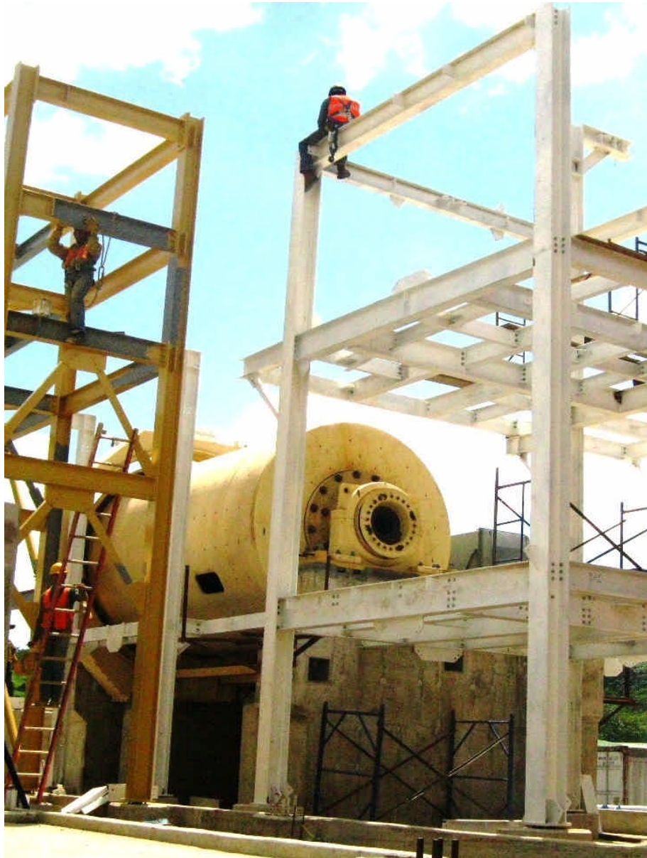
ballmill and piperack erection
