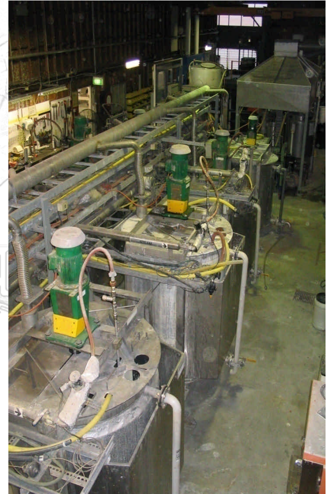
Albion Pilot Plant, Brisbane
