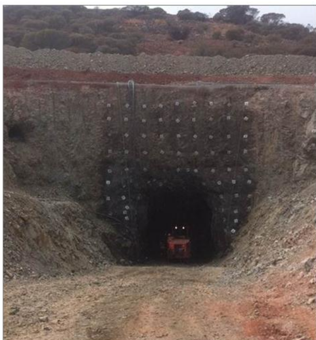
Figure 3: Jumbo entering recently excavated Box Cut and Portal
