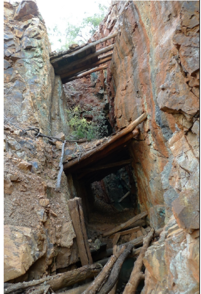
Photo: Silverwood copper mine on the Glentanna project, 2010
