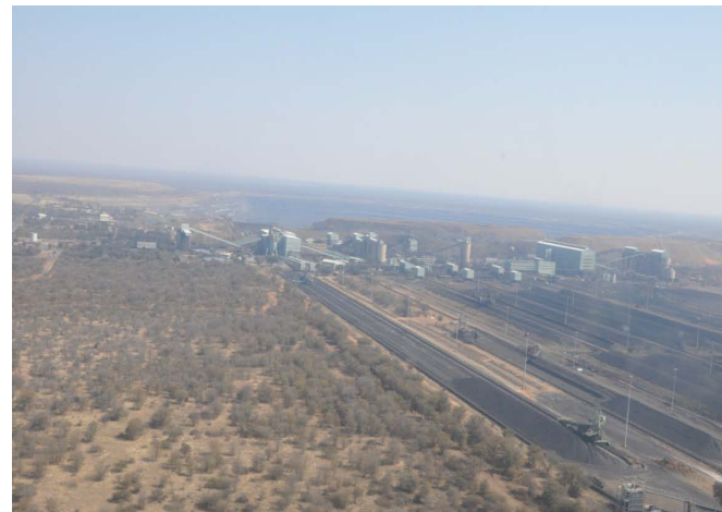
Exxaro Processing Plant
