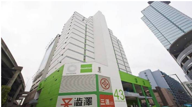
Cargo Consolidation Complex Kwai Chung, New Territories, Hong Kong
