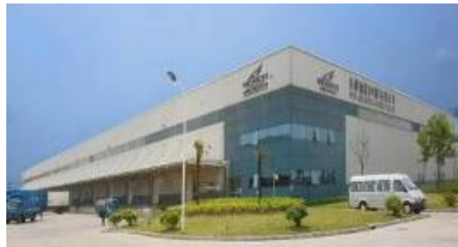
Taopu Industrial Estate Shanghai
