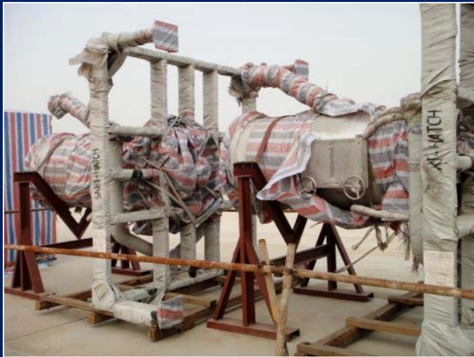
Plant and equipment on site ready for installation
