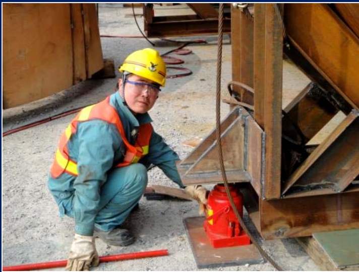
Welding of Calciner kiln shell
