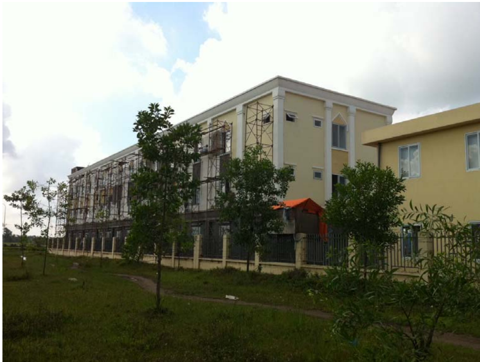
Rear view of main office building
