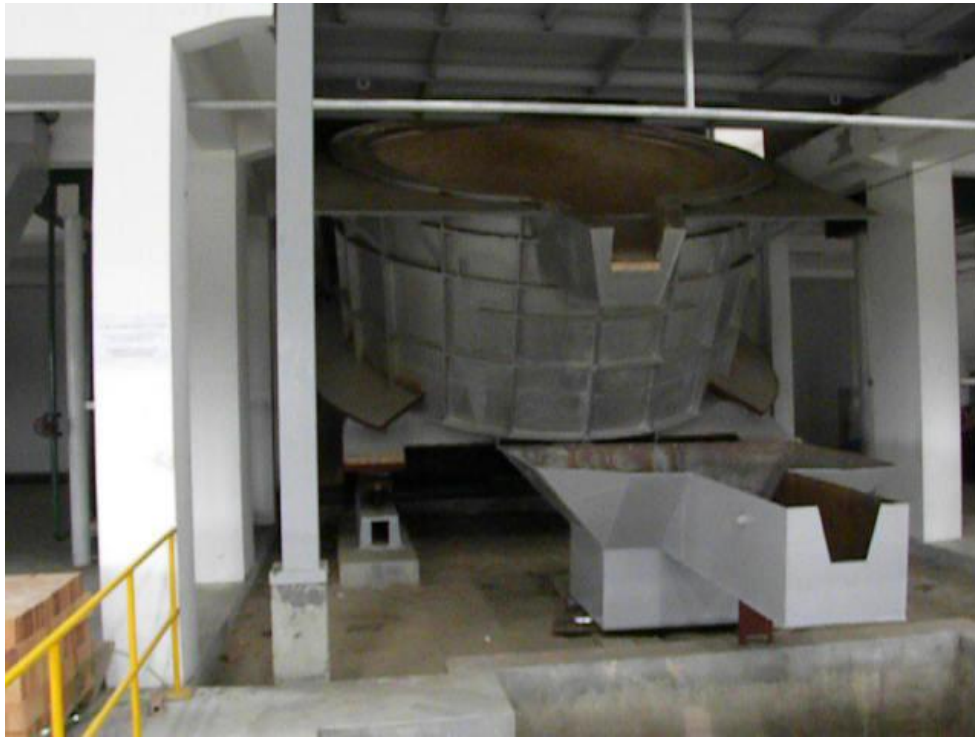
Mechanical (cold) commissioning of furnace tilting hydraulic system
