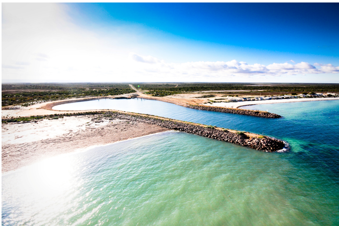
Figure 1: Existing Lucky Bay facility
