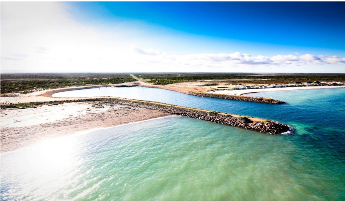
Figure 4: Existing Lucky Bay facility
