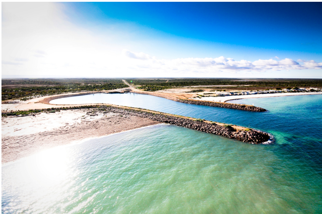
Figure 1: Existing Lucky Bay facility
