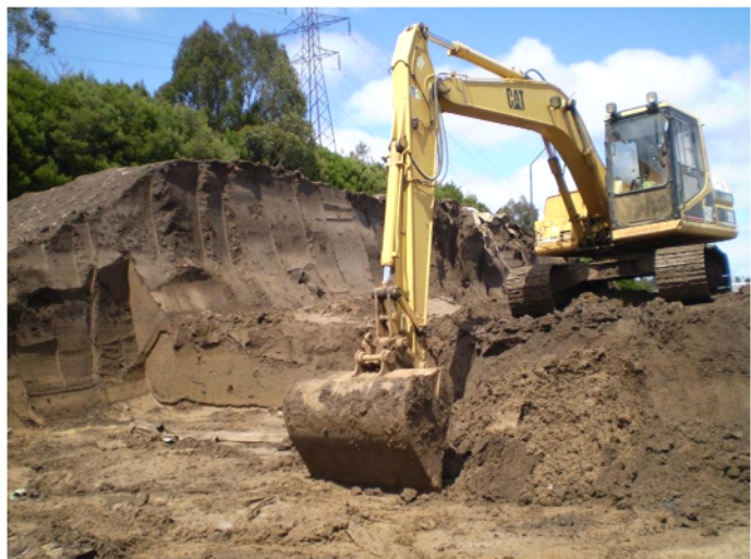
Recovering the EAF dust stockpile at Hellyer
