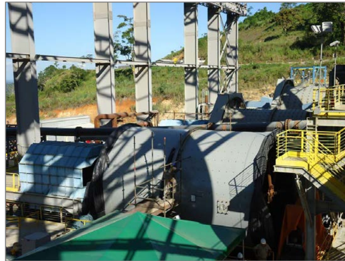
Ball Mill Shell Installed
