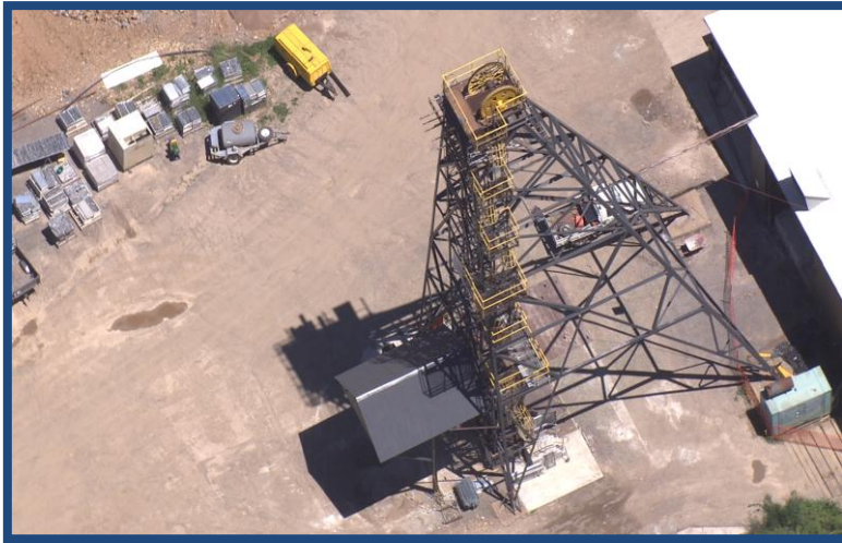
Aerial View of headframe at Morning Star
