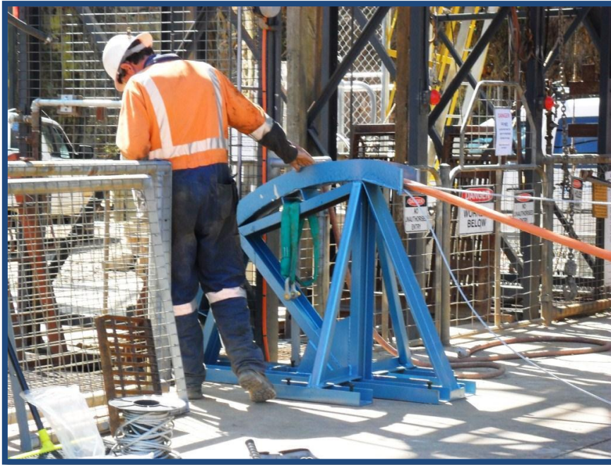
1000v cable being lowered down the mineshaft
