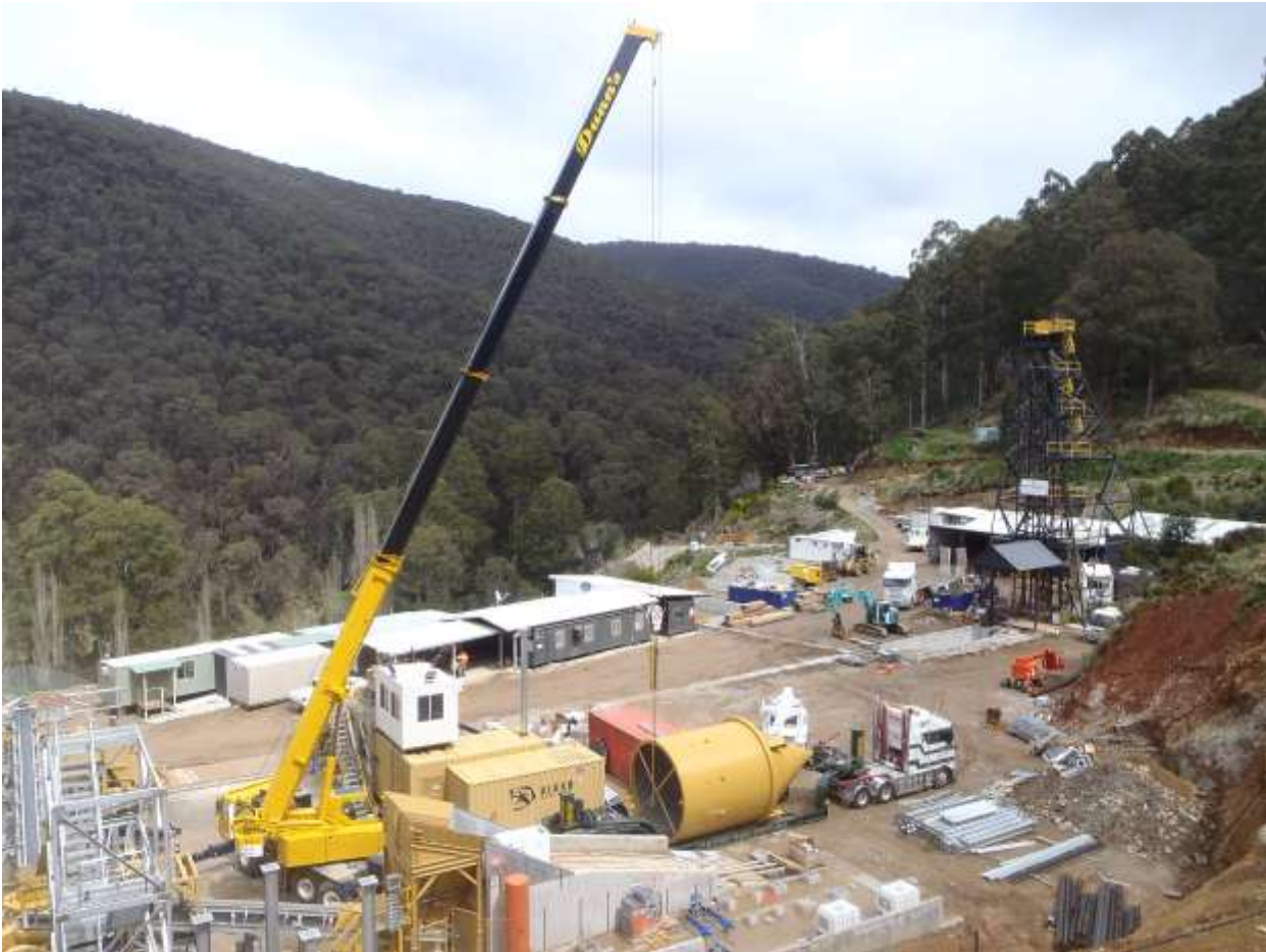
Figure 2: Paste Plant Pachuca being lifted into Position
