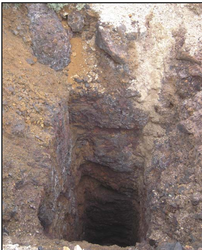
Figure 6: Photograph of historic mine shaft with visible iron mineralisation extending to depth at outcrop 4.
