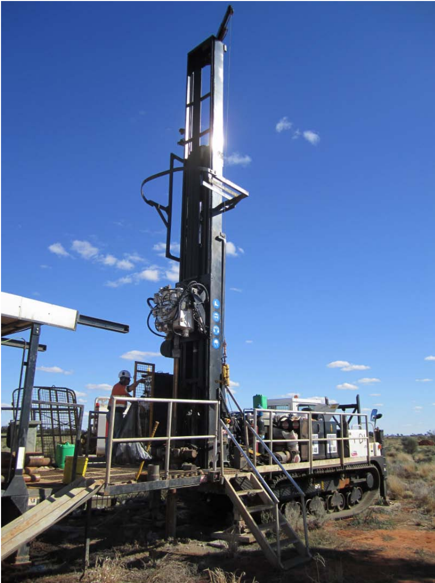
Figure 1: Sonic drilling at Junction Dam – August 2011.
