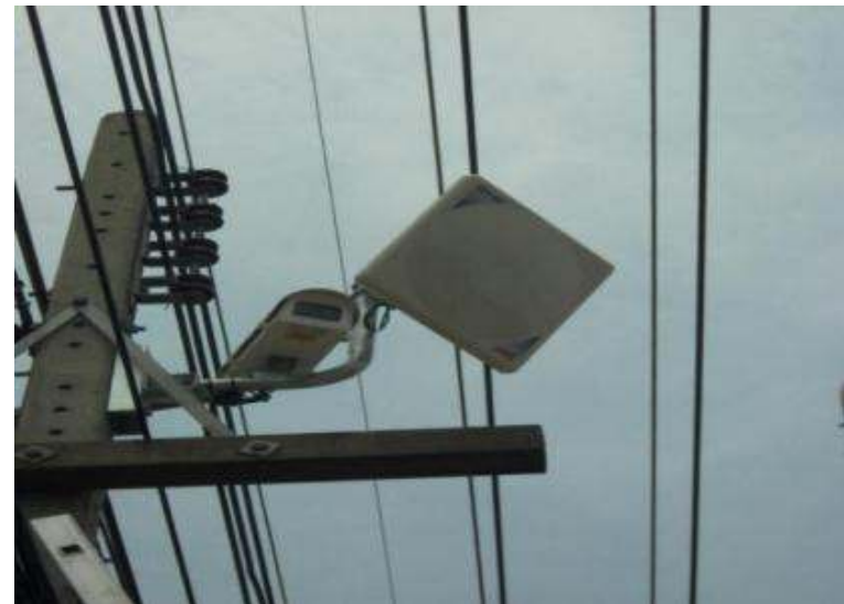
Electrical Post Installation
