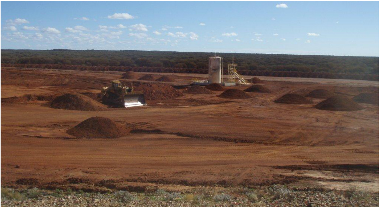
Photo 2. The CAT D11N on the edge of the pregnant solution pond with the flood bund and cyanide tank works in the background.
