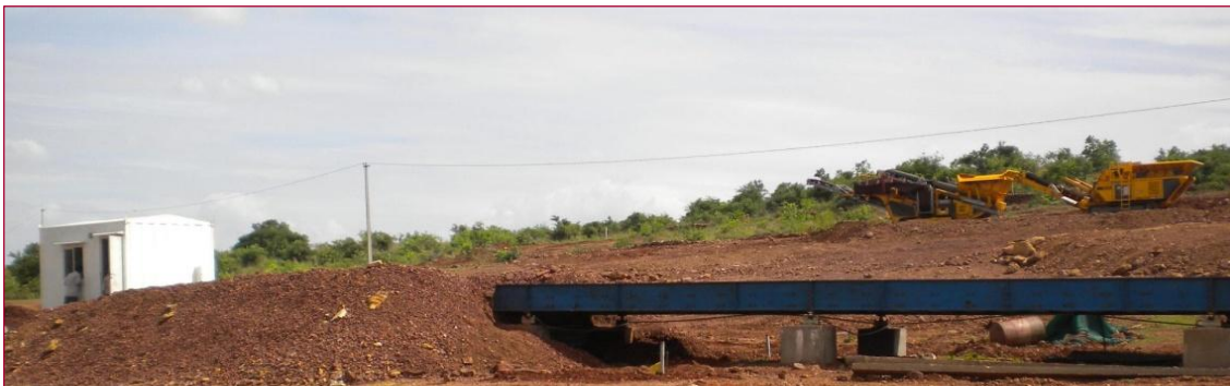
NSL Stockyard facilities, including weighbridge
