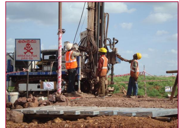
Drilling underway at Kuja
