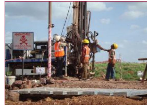
Drilling underway at Kuja
