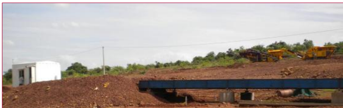
NSL Stockyard facilities, including weighbridge
