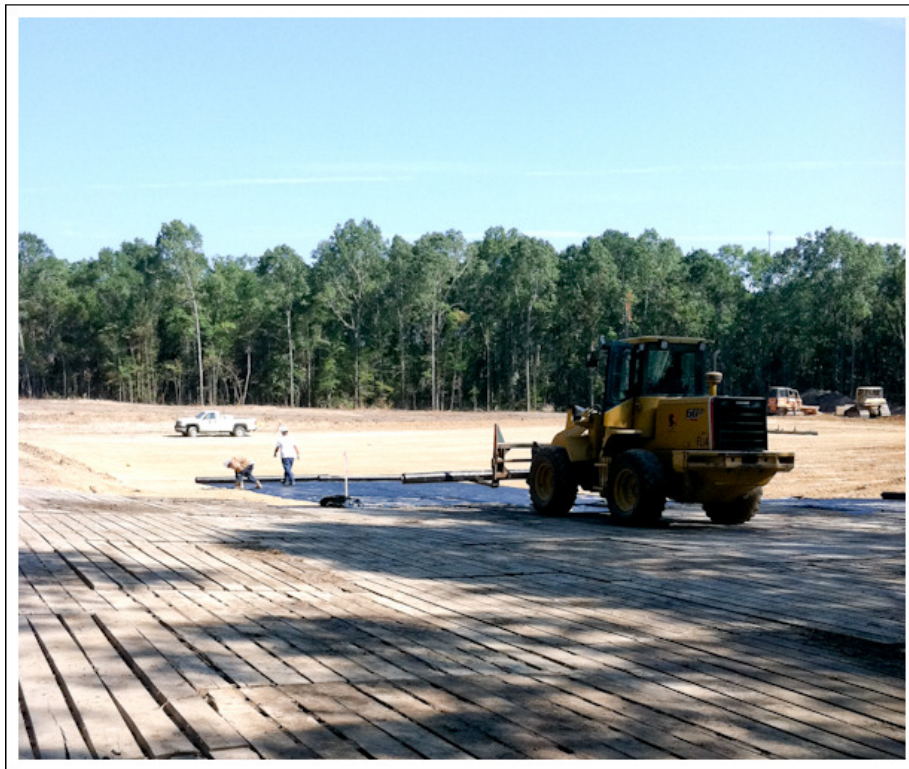
Well # 1 Location site work in progress.
