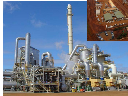
BHP's acid plant at Ravensthorpe, WA (below)
