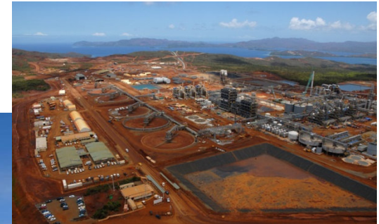
Goro nickel plant in New Caledonia (above)
