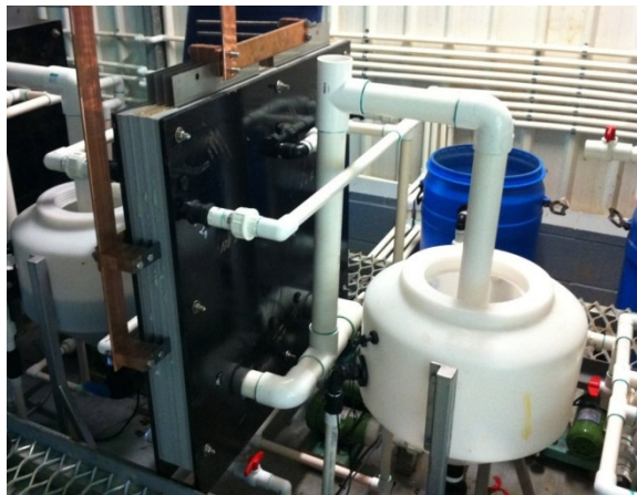
The pilot plant (above) is currently in its second-last iteration
