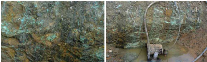
Mt Norma wall of super vat showing the copper oxide mineralisation discovered while constructing the new vat
