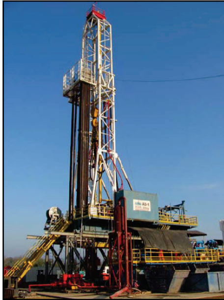
AD-1 Drilling Rig
