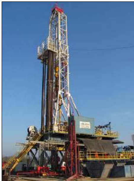
AD-1 drilling Rig
