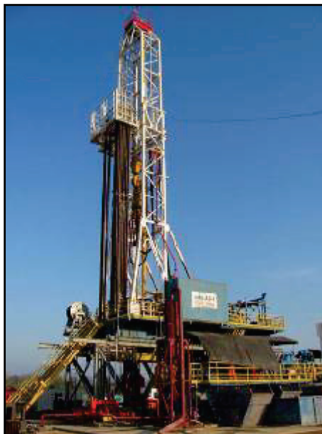
AD-1 drilling Rig
