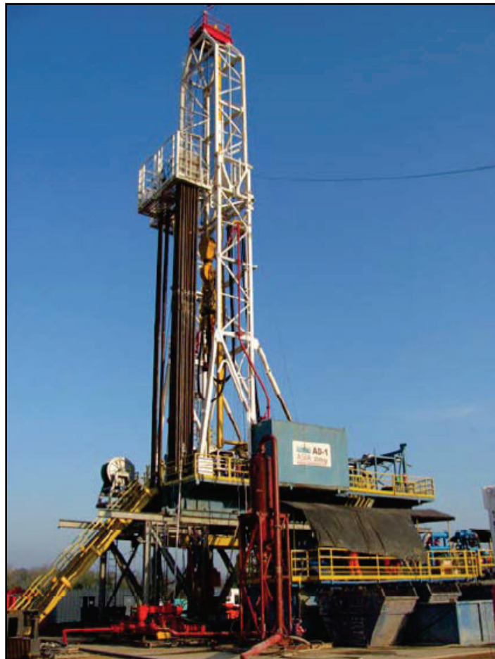
AD-1 drilling Rig
