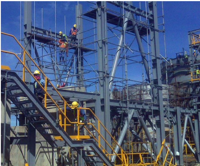
SAG mill platform and cyclone tower steelwork.
