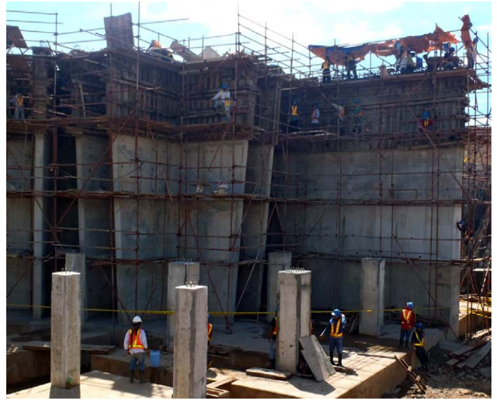
Crusher station foundation and supporting structure.
