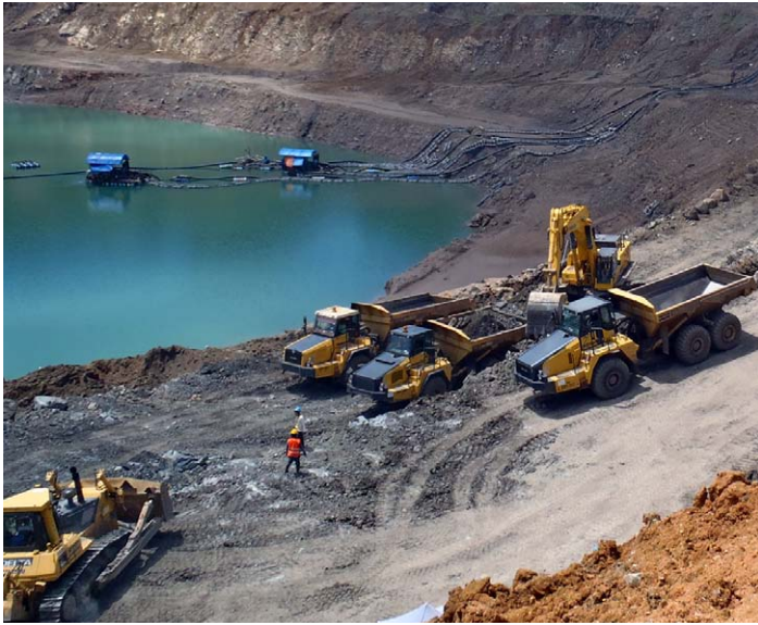
Open pit cut back activity with pit dewatering in background.
