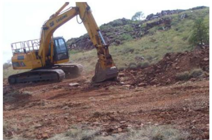
Figure 5 – Excavation and re-fill of costeans showing disturbance to available surface exposure
