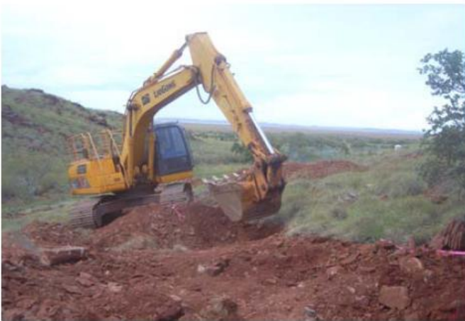
Figure 5 – Excavation and re-fill of costeans showing disturbance to available surface exposure
