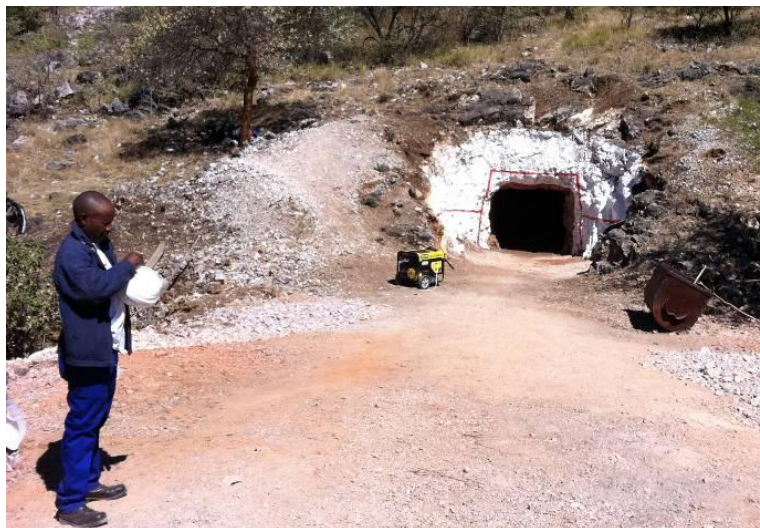
Figure 3 - Rehabilitation of the historic workings adjacent to Kaskara will provide underground access to mineralisation and drill collar sites.
