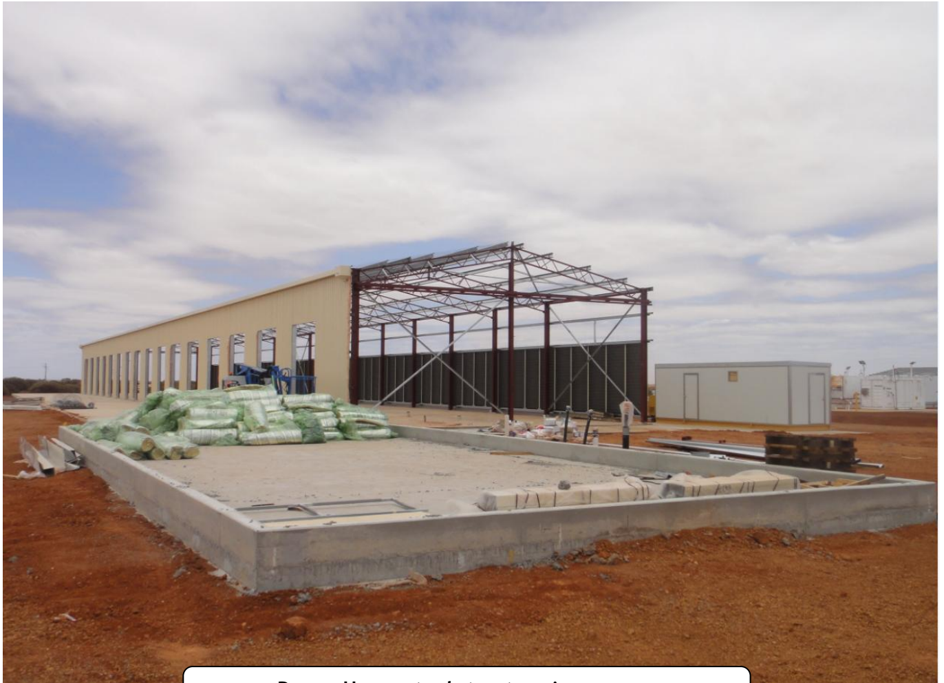
Power House steel structure in progress
