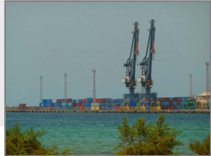
Existing port of Massawa, Eritrea.
