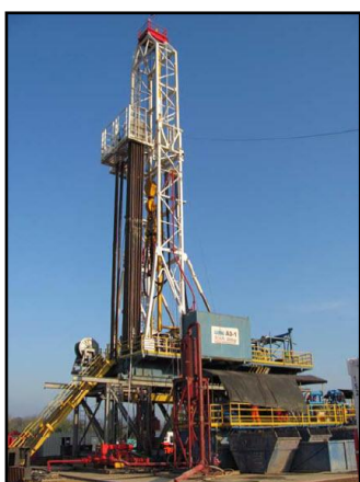
AD-1 Drilling Rig
