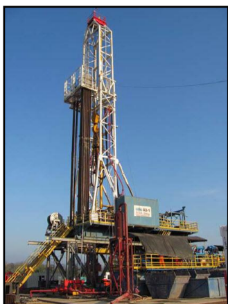
AD-1 Drilling Rig
