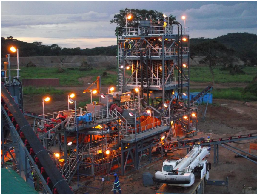
Kipoi Heavy Media Separation Plant ready for commissioning.
