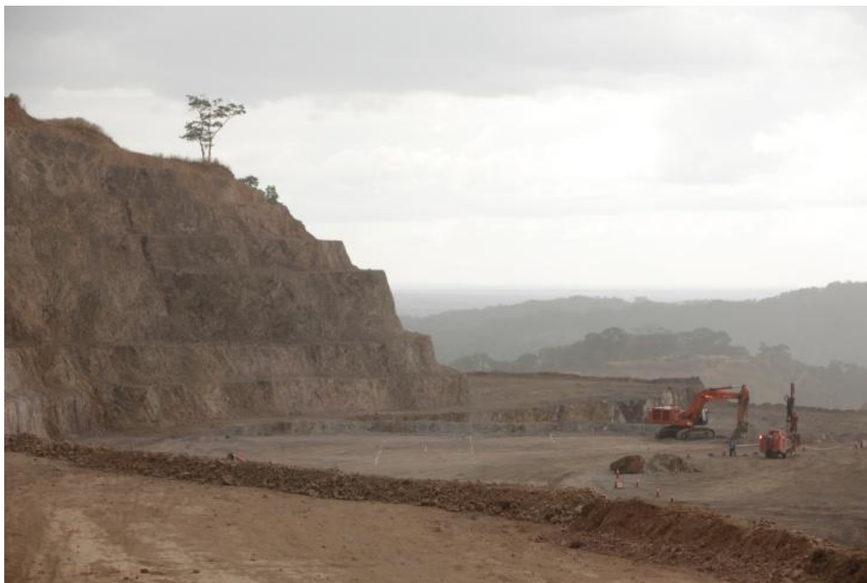
Kipoi mine – 31 May 2011
