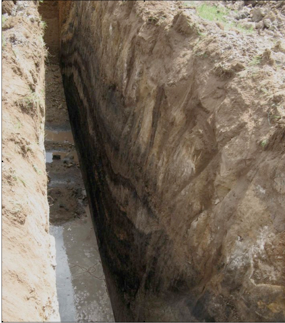
Figure 1: Trench 01 showing coal in base of trench
