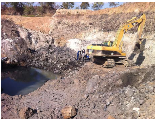
Inspection of the pit following blasting
