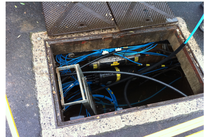
New Vocus Fibre being Installed June 2011
