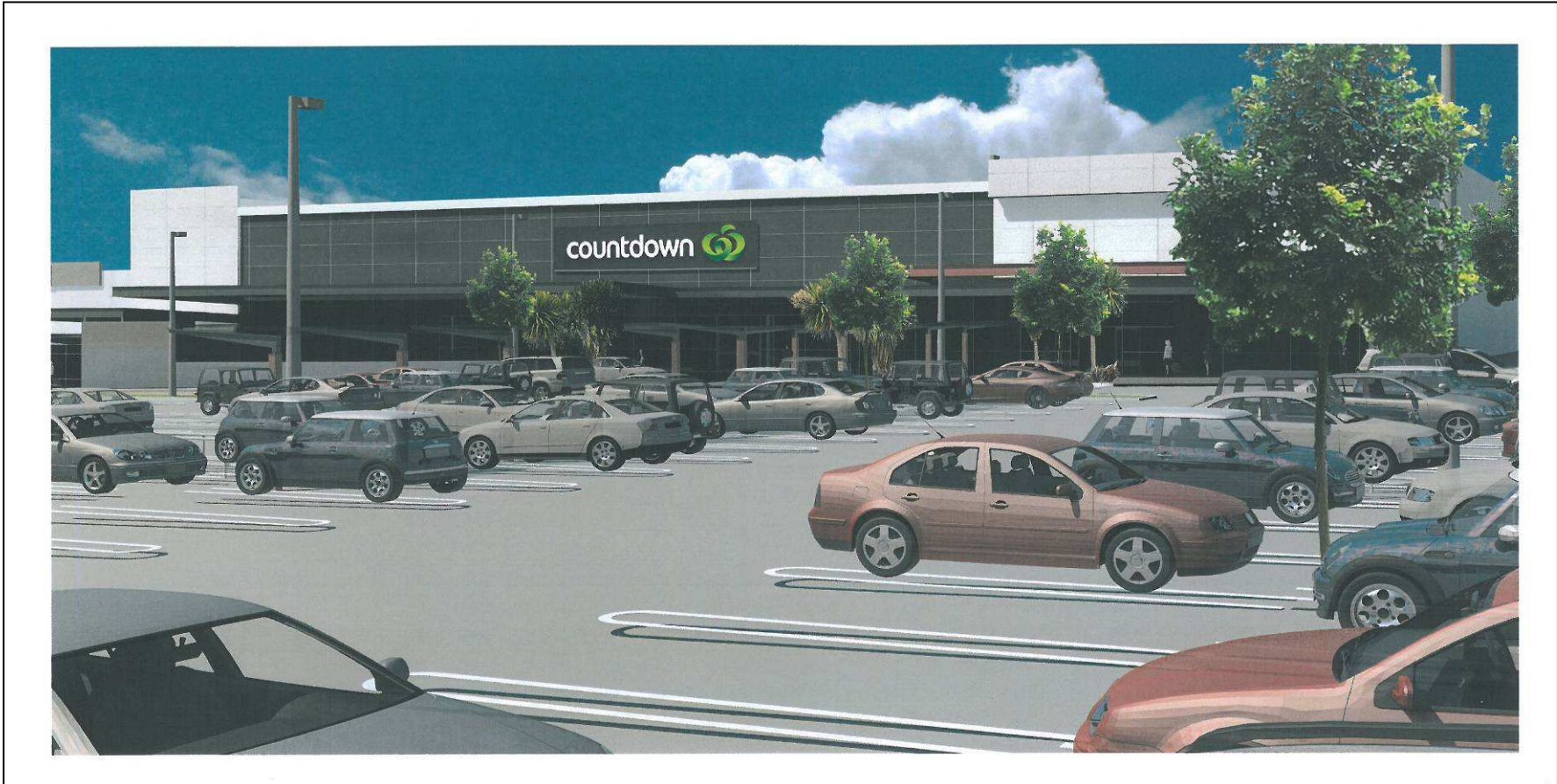
Co-anchor Countdown Supermarket at 4200m 2 GFA
