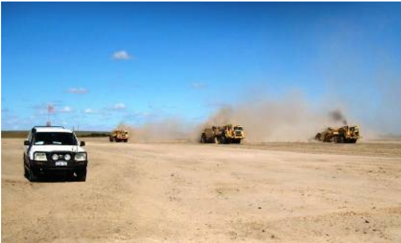
Three scrapers stripping topsoil at Mosso Farm evaporation pond
