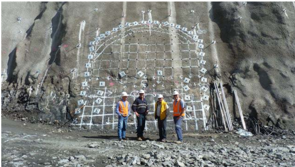
Photograph of portal position for Spotted Quoll decline mine, prior to blasting on 20 th April
