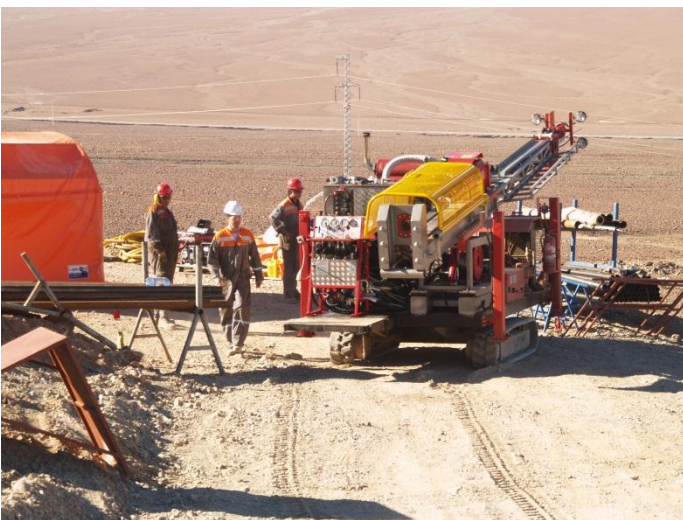
Figure 3 – Drill Rig Set-up at the Nany Project, Atacama Desert, Chile
