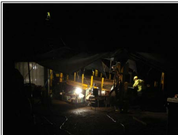
Night time drilling at Anthony
