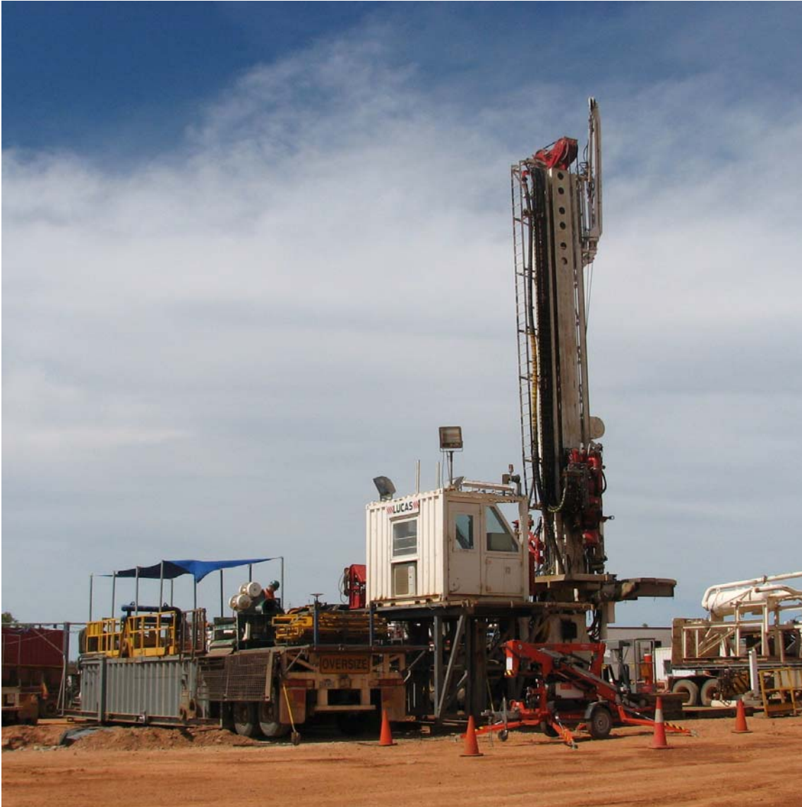
Figure 3: Drilling Rig on Cow Lagoon #1 Well
