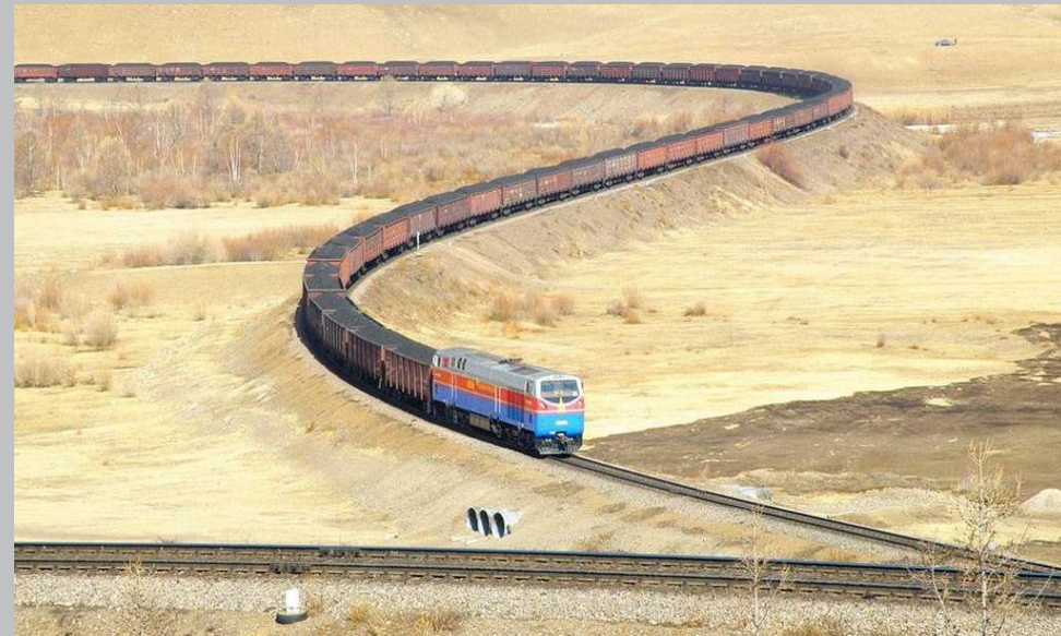
Trans-Mongolian Railway, coal from Baganuur coal mine
