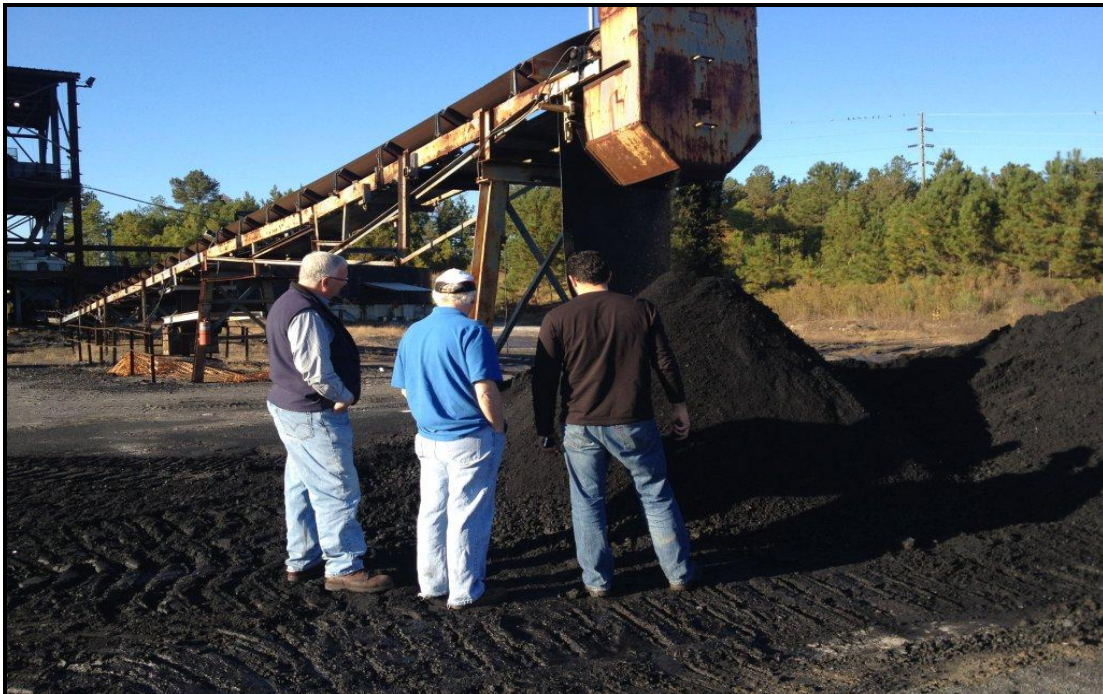
Figure 2. Inspection of clean coal produced from Kodiak Preparation Plant
