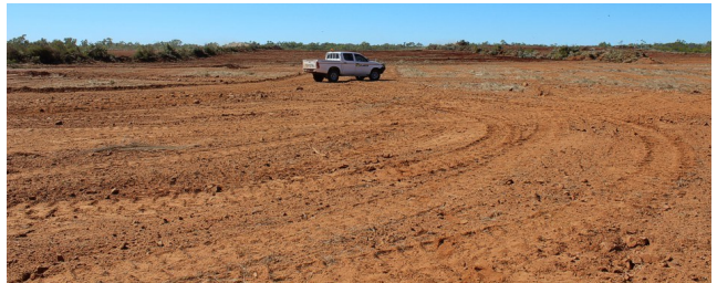
Figure 23: Initial scrape-back of Plant site - all machinery owned 100% by CuDeco
