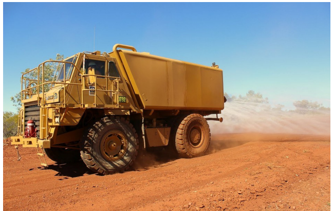
Figure 21: Dust suppression on major access road construction - all machinery owned 100% by CuDeco
