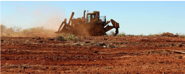
Figure 22: D11 preparing Plant site - all machinery owned 100% by CuDeco
