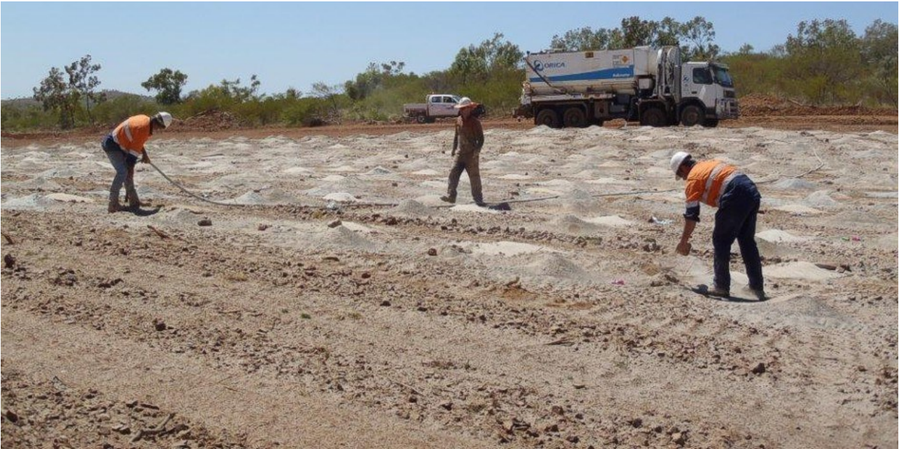
Figure 2: Charging Blast Holes with bulk explosives and Priming.
