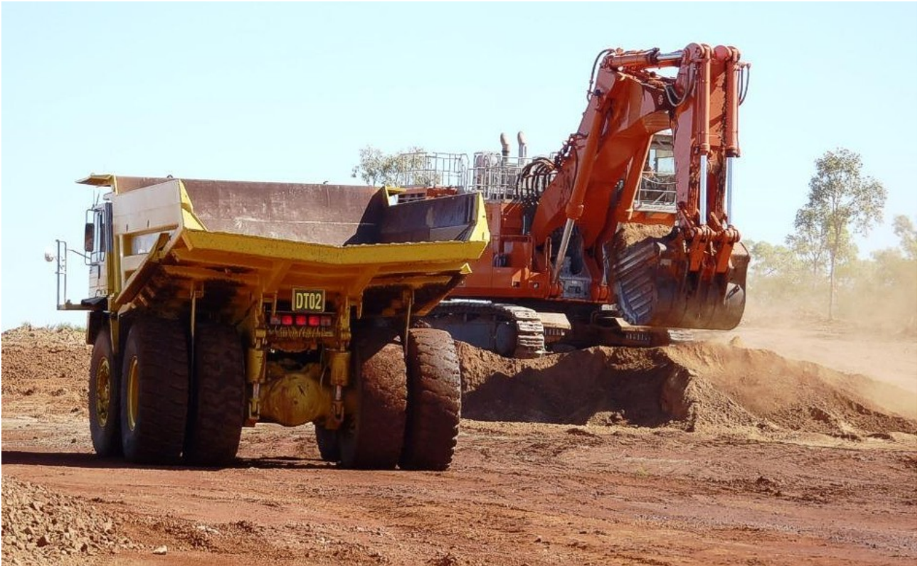
Figure 28: Dump truck and excavator working at Morris Creek Diversion Channel excavations.
