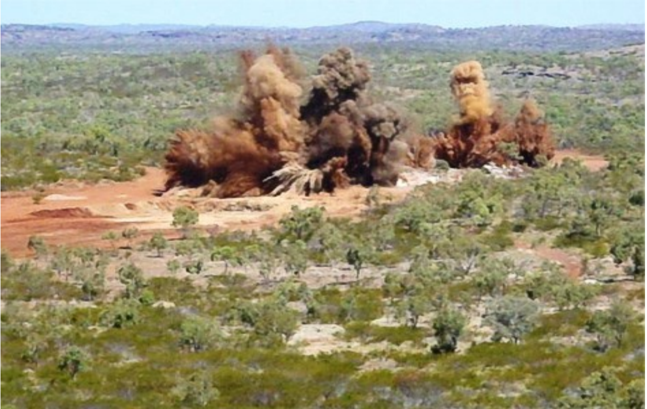
Figure 34: Second “shot” of the project - during construction of the Diversion Channel
