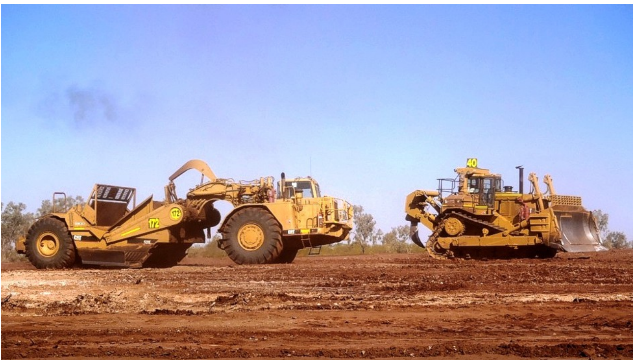
Figure 29: Scrapers levelling and removing clays at the Process Plant site.
