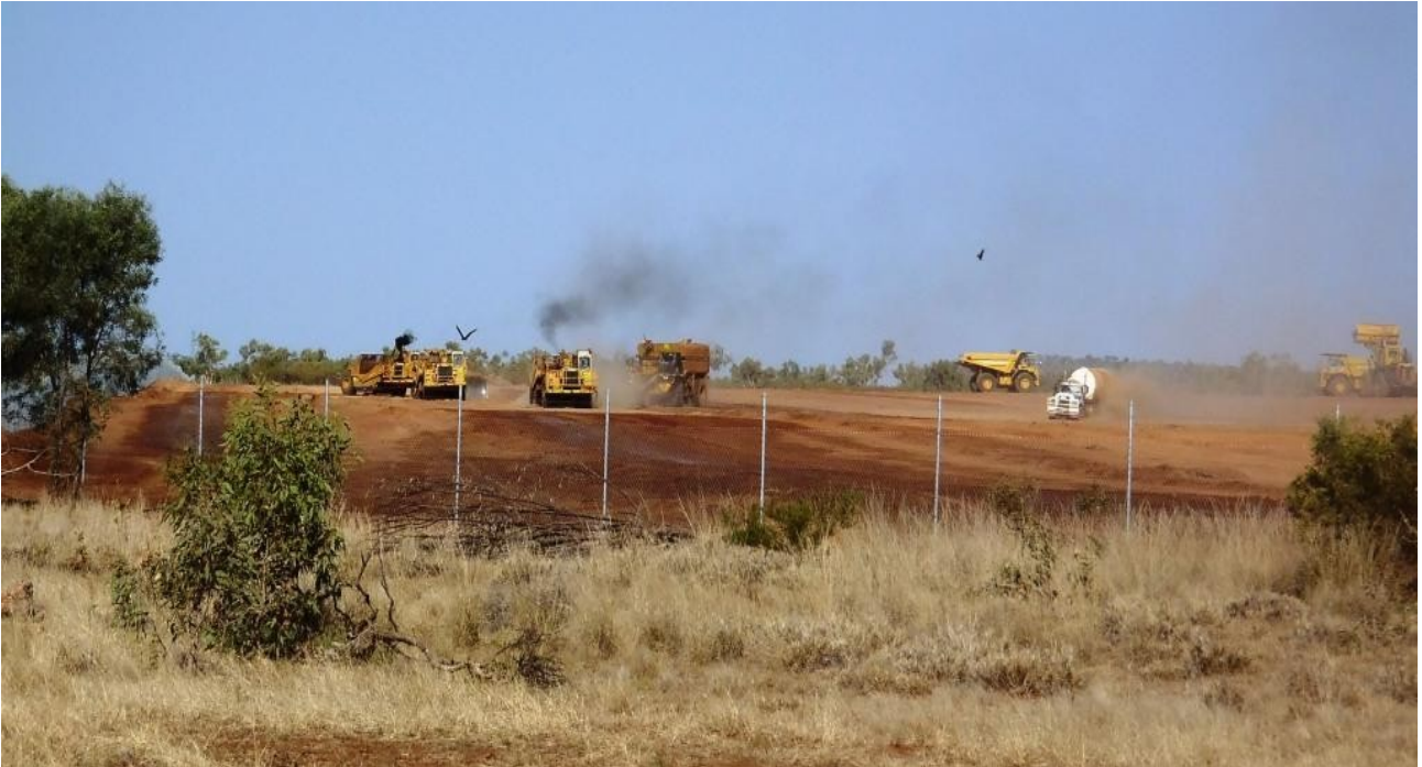
Figure 35: Significant activity at the Tailings Storage Facility (TSF) - removal and storage of organic material & topsoil for use in later rehabilitation, and laying of clays to base of tailings cell 01.
