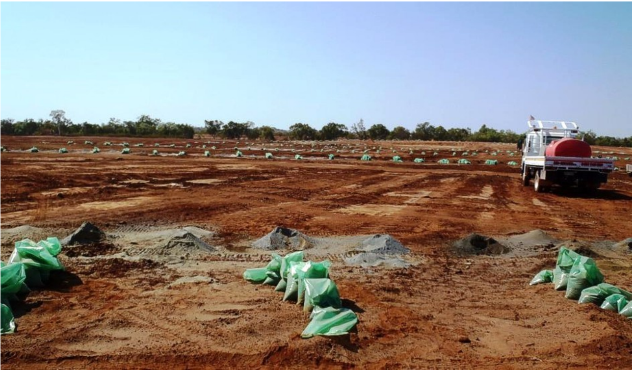
Figure 27: Sample bags remain on the various bedrock lines over the Las Minerale starter-pit area. Numerous zones of mineralisation have been identified within the predominately “free-dig” zone in the planned pit area, additional to identified ore zones, that will be stockpiled
