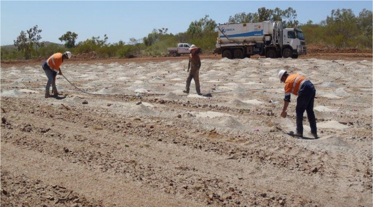
Figure 9: Charging Blast Holes with bulk explosives and Priming.
