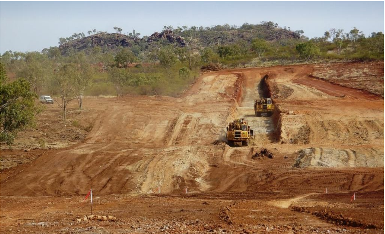
Figure 31: Morris Creek Diversion Channel Dam Wall - structural excavation and site preparation.
